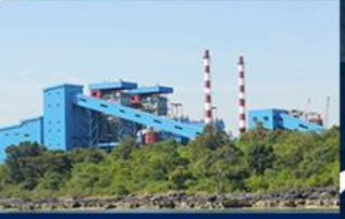
PLN Power Station
