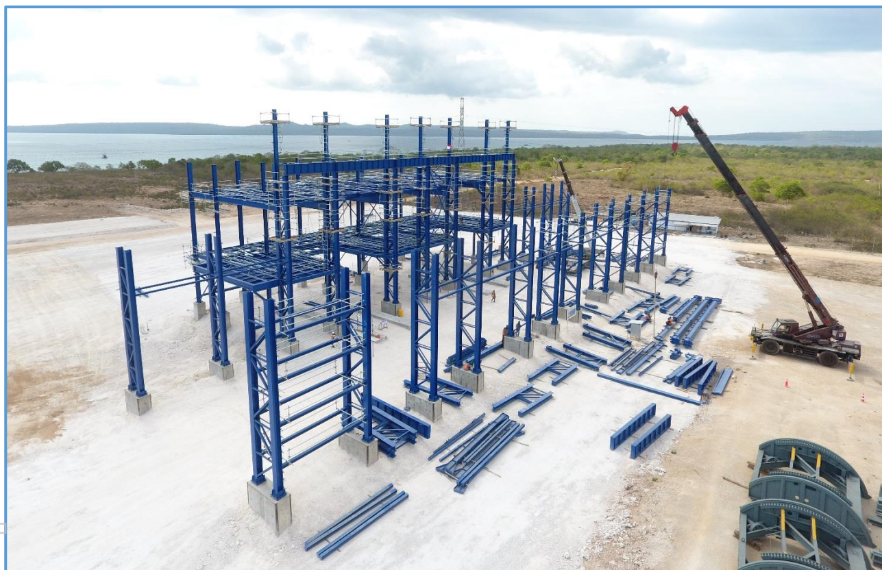
Figure 1: Latest development progress at the Kupang Smelting Hub Facility
